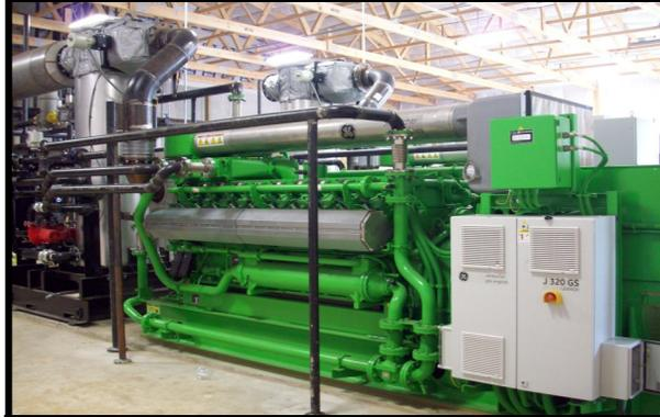
Bio Town® Ag's Energy Center, located just north of the Town of Reynolds, utilizes the manure generated from Bio Town® Ag's cattle feedlot and swine facility along with other organic products for processing in an anaerobic digester to generate methane gas. The gas is then used to power internal combustion engines to generate 3 megawatts of electricity per hour, which supports the Bio-Town® USA initiative of developing a community that is self-sustainable using bio-renewable resources.
